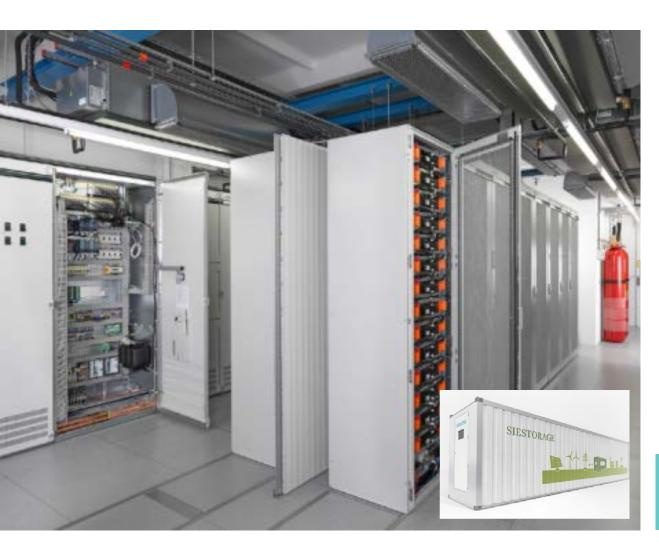
Modular energy storage system based on cutting-edge power electronics and Li-ion batteries:
